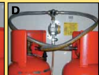
Picture shows a Truma regulator upgraded to a manual changeover with a 01-1630 and using two propane 0.75 meter Stainless hoses. Note how the hoses cross preventing unnecessary kinking and twisting.
