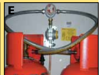
Picture shows a Truma regulator upgraded to a Auto changeover with a 01-1755 and using two propane 0.75 meter Stainless hoses. Note how the hoses cross preventing unnecessary kinking and twisting.
